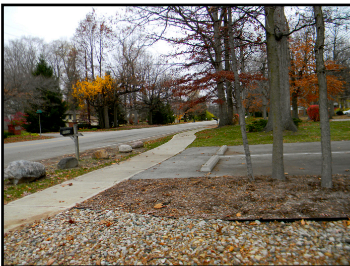
Figure 2:. Fragmented sidewalks near JCC property.
